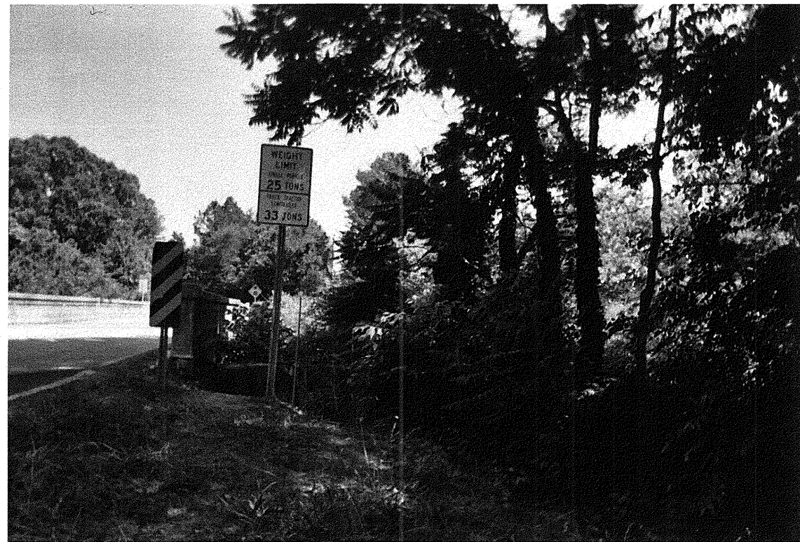
Photograph 1 – View Approximately 15' Rt. of -L- Looking Upstation from EB1-B
