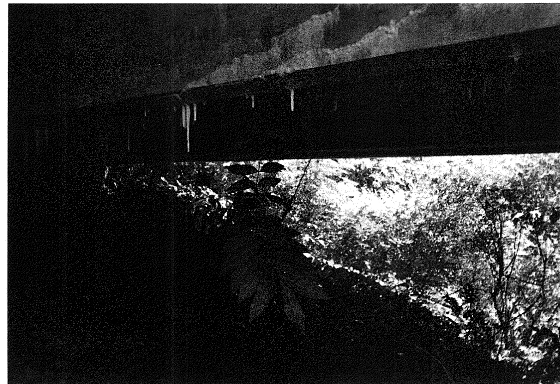
Photograph 7 – View Left to Right Across Bent-2
