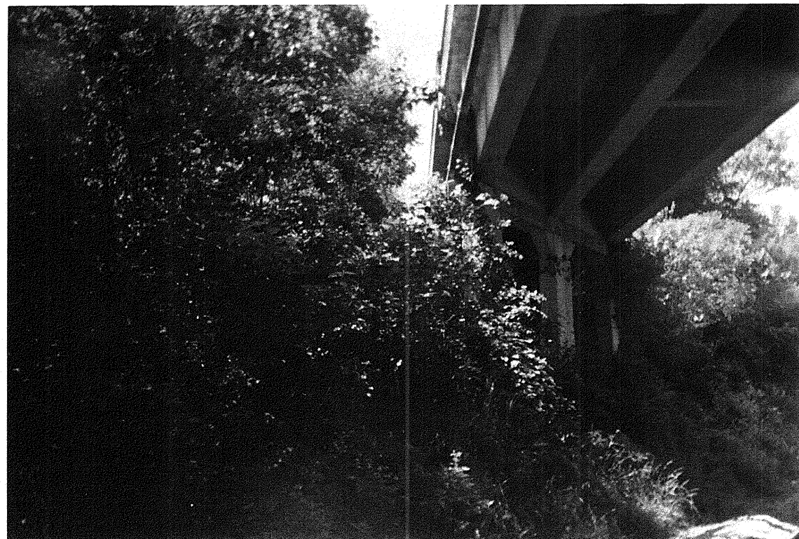
Photograph 2 – View Approximately 15' Right of -L- Looking Downstation from Railroad
