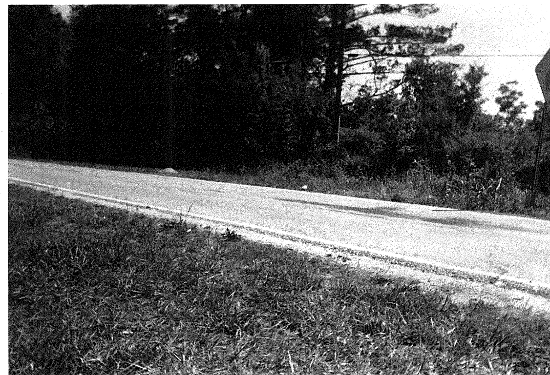
Photograph 8 – View Left to Right Across End Bent-2
