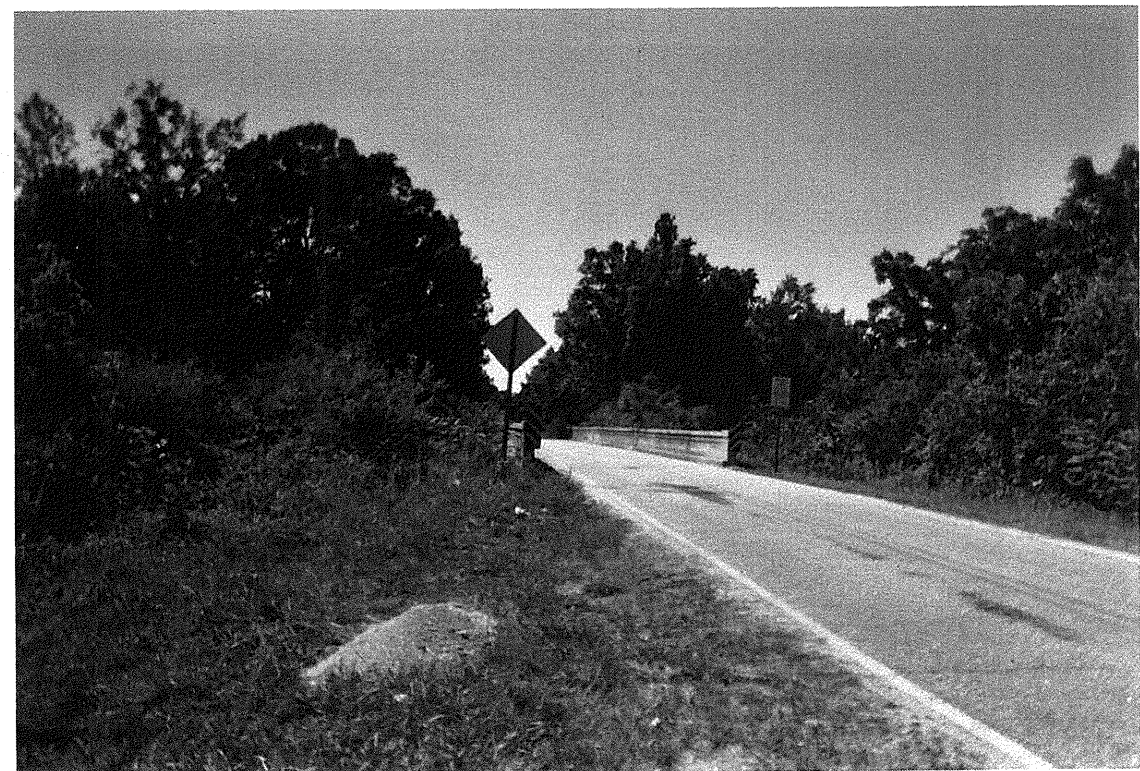
Photograph 4 – View Approximately 15' Rt. of -L- Looking Downstation from EB2-B
